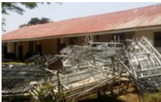
Unnecessary equipment was dumped in the yard
