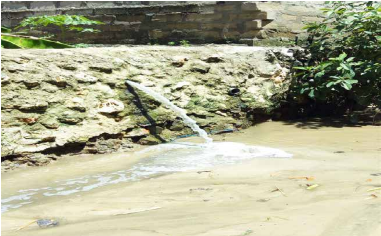
Figure 92: Discharge of wastewater from an industry to the Mlalakuwa River
